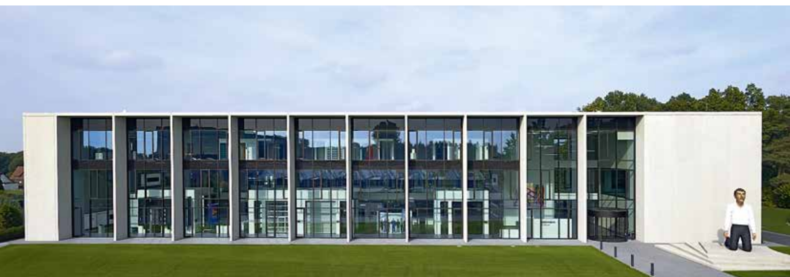
The new Hörmann training and exhibition centre at the headquarters in Steinhagen.
